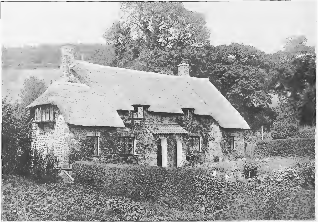
A HOUSE ON THE ROAD FROM MINEHEAD TO PORLOCK
